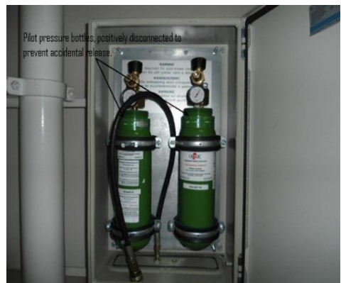
Release cabinet with detached hose for positive action release
